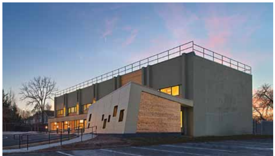
The warehouse was transformed into a handsome, energy efficient building.
